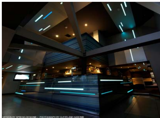
Light Tape installed at Bar 195 Epping
